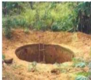
Figure 10: Pit for the tank construction
