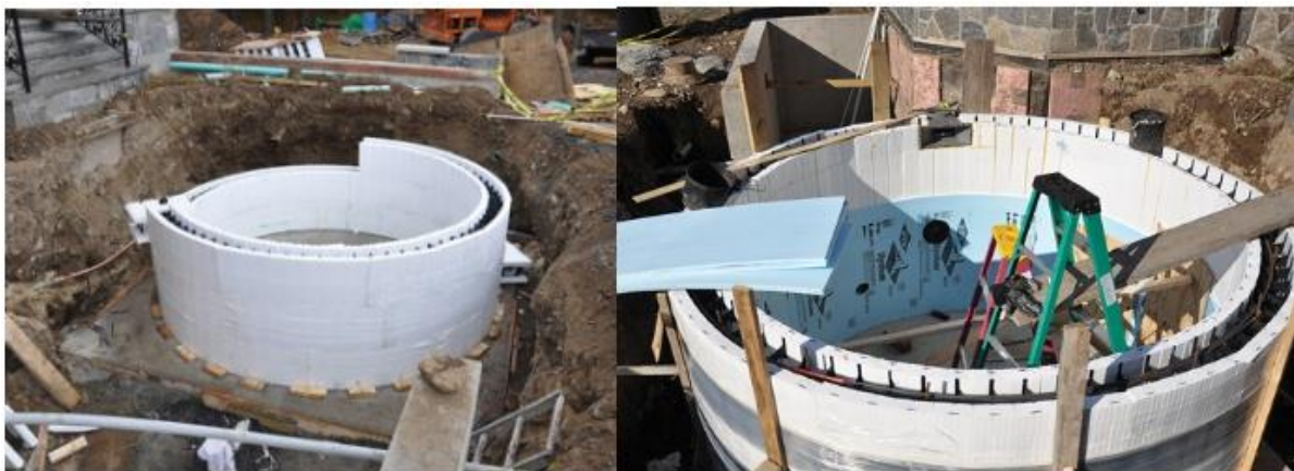
Figure 7: Foam concrete water tank construction
