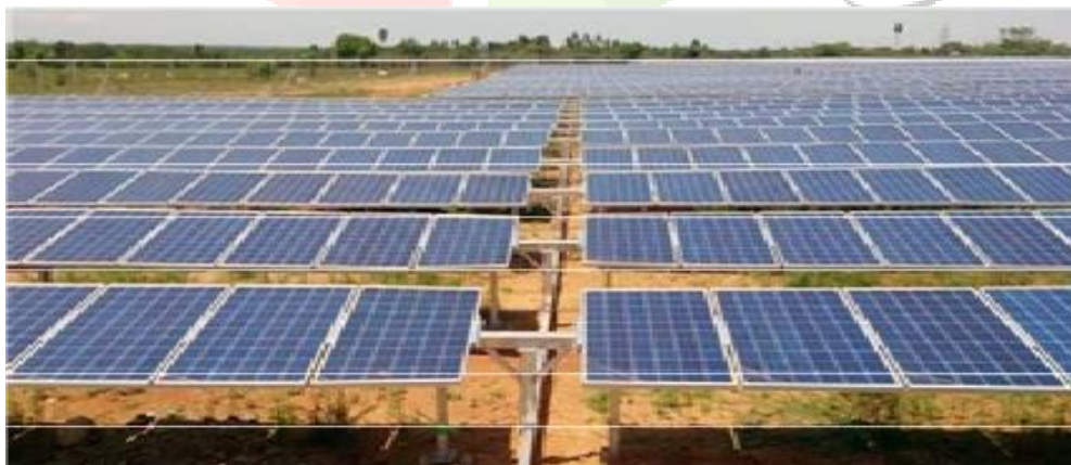
Fig 3 Horizontal Single-Axis Solar Tracker (HSAT)
