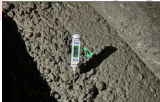
Fig.09. Concrete temperature at site
