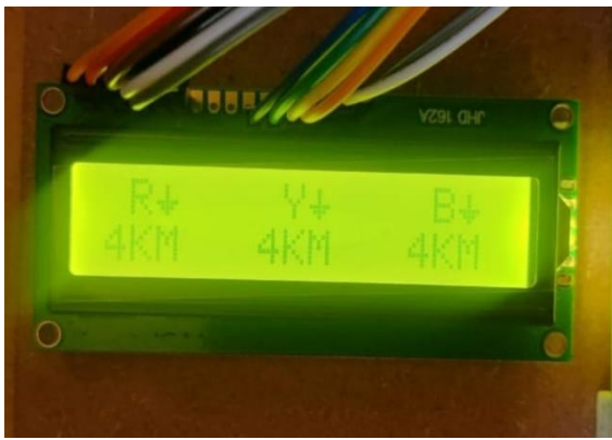
Fig.4 : 4 km switch is OFF in all three lines (R,Y,B)
