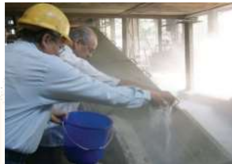
Fig 1.8 Transfer of aggregate
