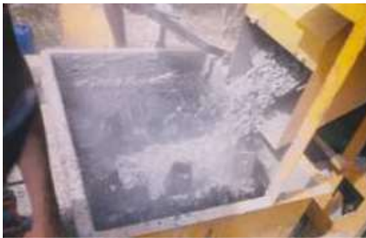
Fig 1.7 Transfer of aggregate
