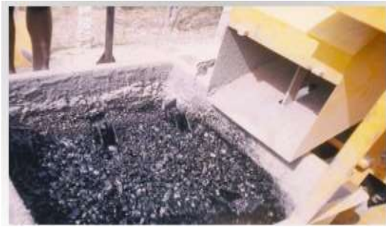
Fig 1.11 Aggregate plastic bitumen mix
