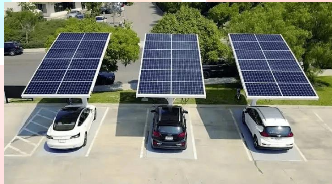
Fig-1 solar based EV wireless station
