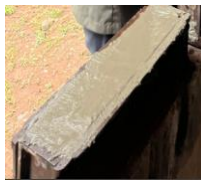
Fig. 8 Beam casting
