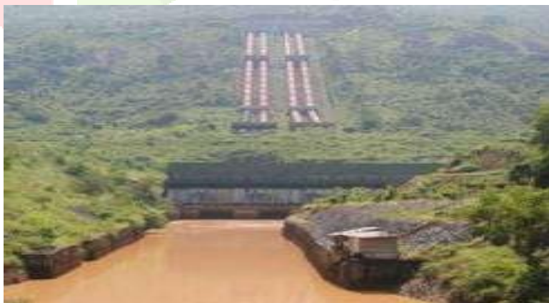
FIG-3 : SHOWS THE OUT LET TUNNEL WITH WATER FOR IRRIGATION
