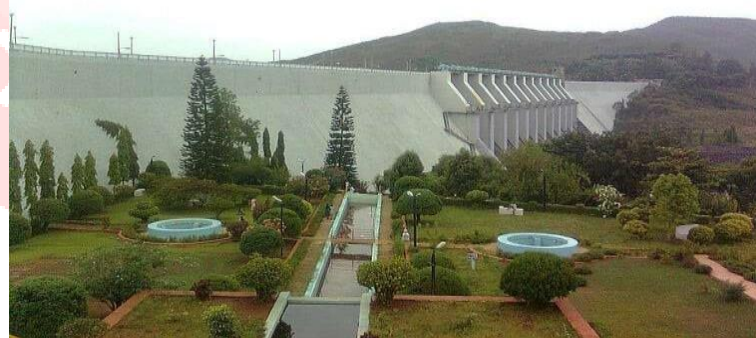
FIG-1 DAM WITH 11 SPILLWAYS
