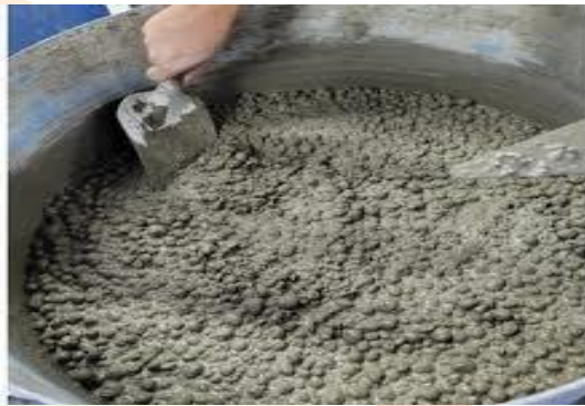
Fig 1: Mixing of Concrete with LECA Aggregates
