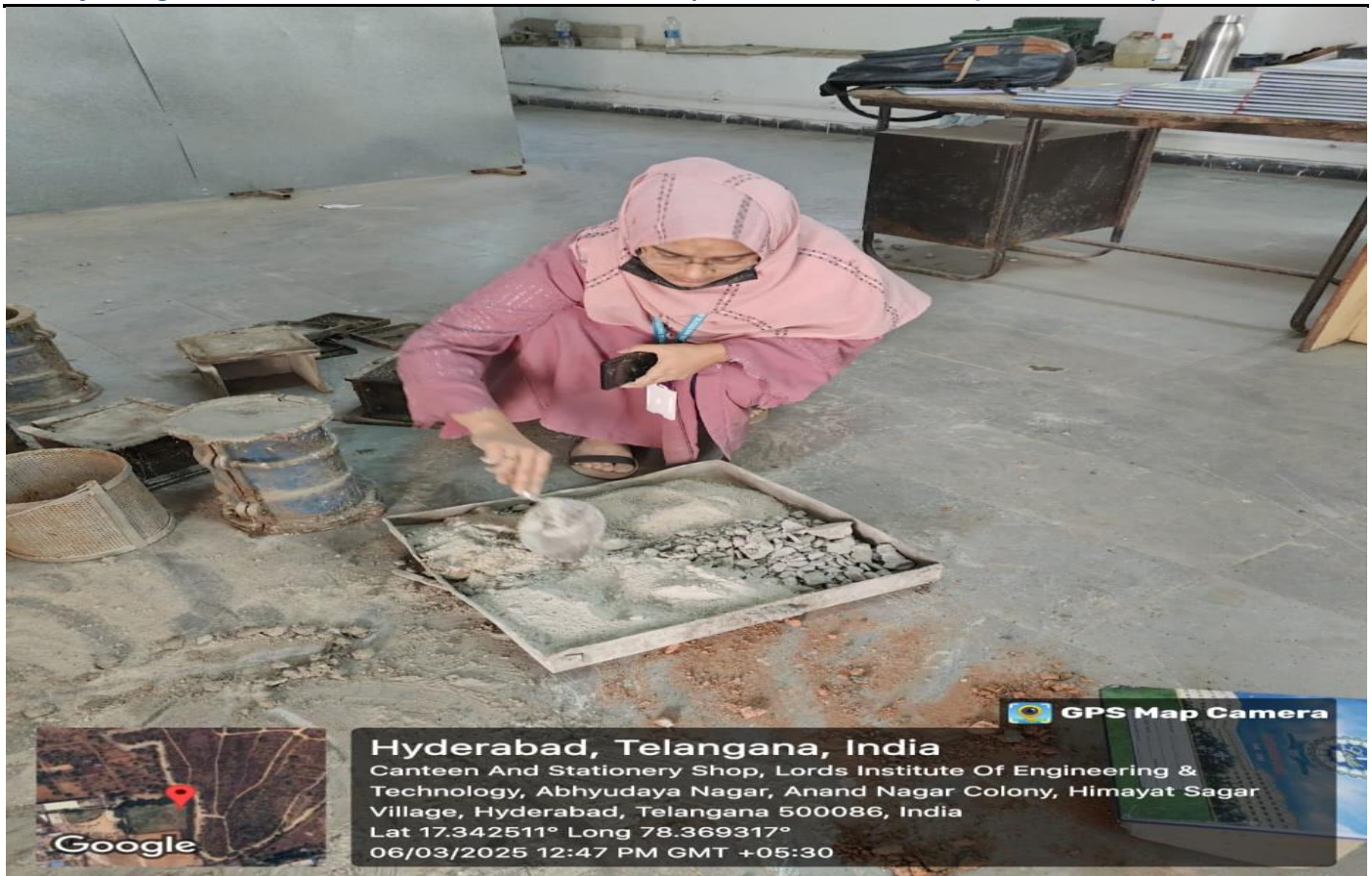
Figure 3.4 Mixing of concrete
