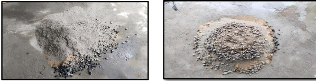
Fig (1): Concrete Mixing
