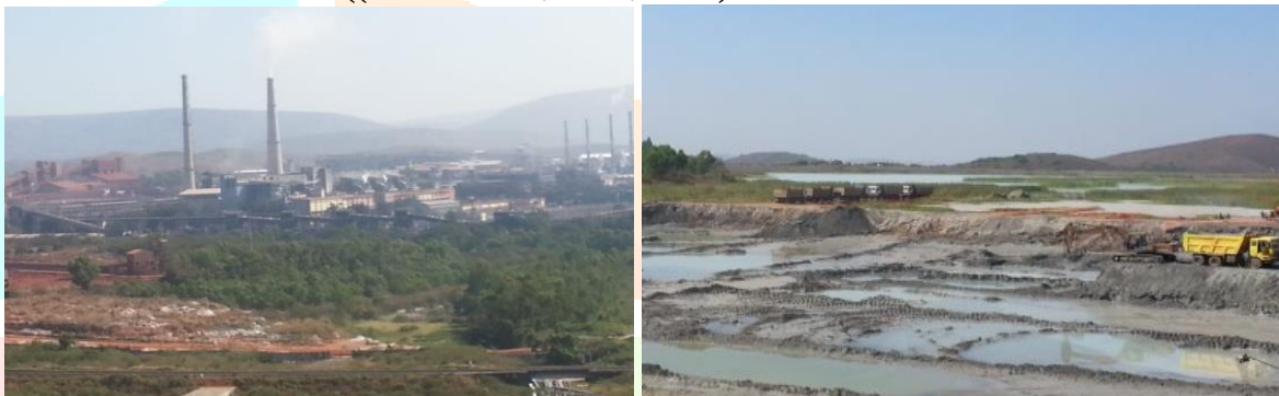
(Photo- Industry & RM Pond down stream area showing wastes and leaching of waste)
