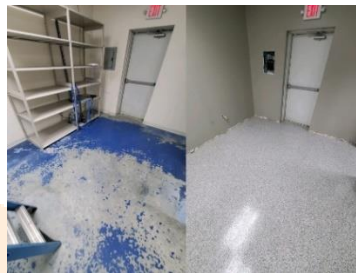
Figure 5: View of the Office area (Port of Houston)
