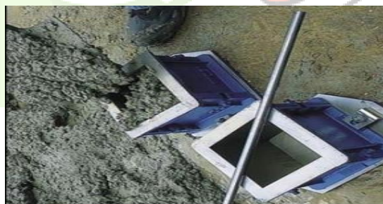
Fig.3 Placing, Compacting, and Finishing
