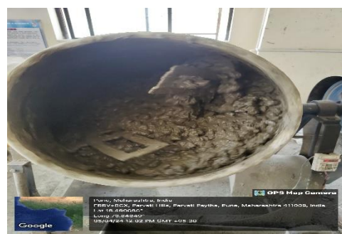
Fig 2: Machine Mixing of Concrete
