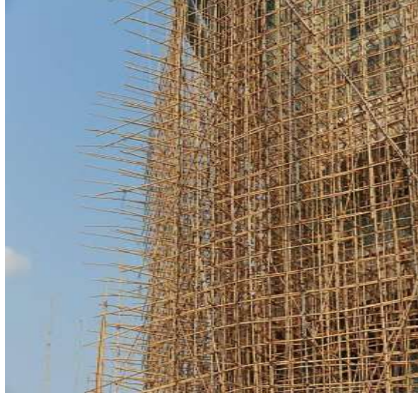
Figure 18 Bamboo scaffolding
