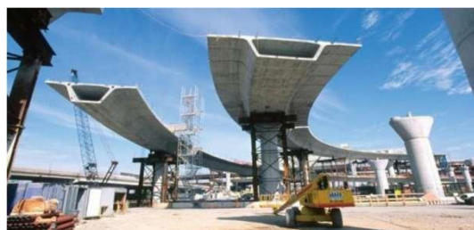
Figure 1.1 Box Girder Bridge
