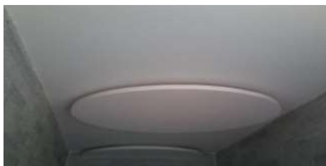
Figure 23-False ceiling with gypsum board in concrete roofed structure
