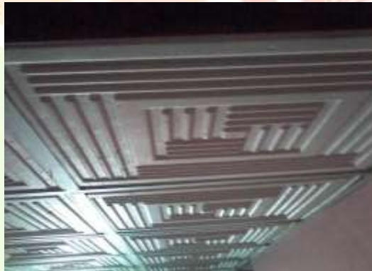
Figure 15–Thermocol false ceiling below concrete roof in a building
