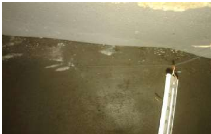
Figure 27 – Bonding thermocol below concrete roof
