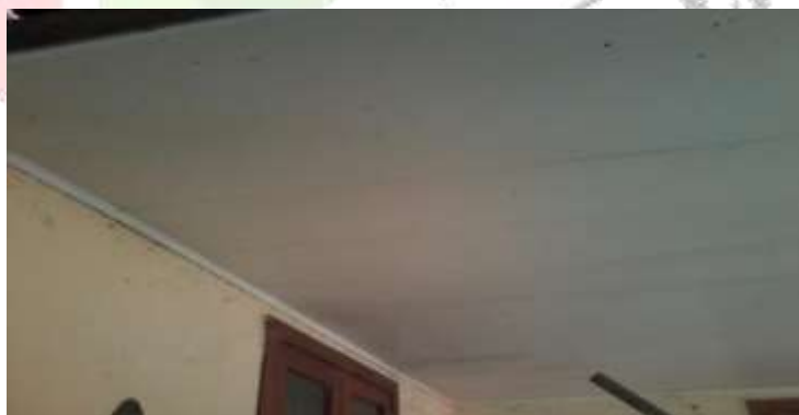
Figure 19 - PVC false ceiling below concrete roof
