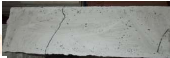
Top view of crack pattern for 50mm thick panel
