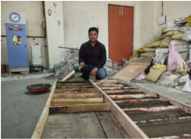
Top view of crack pattern for 20mm thick panel
