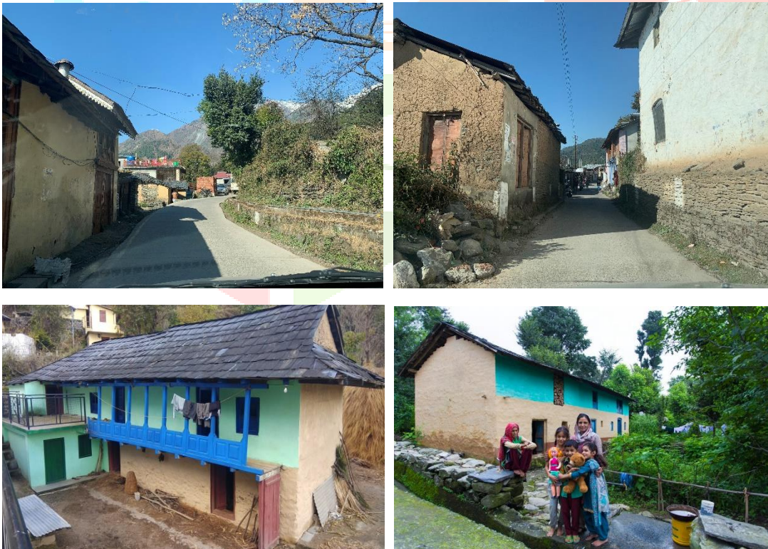
Fig2 : images showing various vernacular material used for construction in villages of dharamshala making development with least impact on environment.
