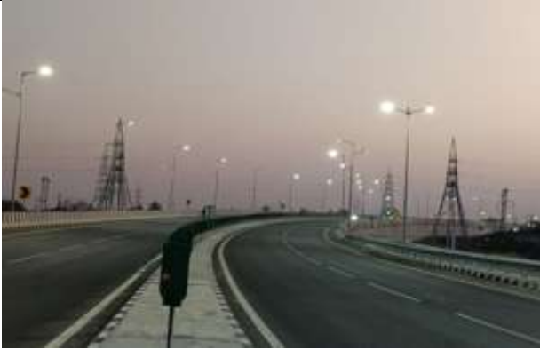
Figure-5 Bridge at Vanthli
