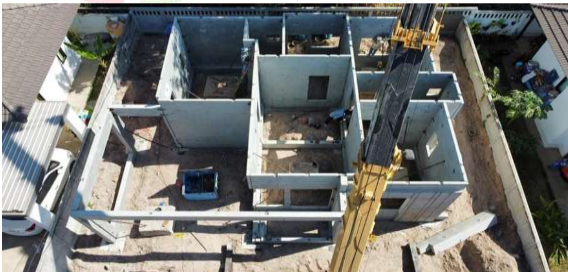
Fig.7 : Precast Panels Under Construction
