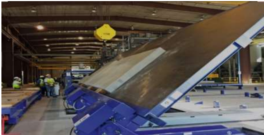
Fig.4 :Demoulding of Precast Elements
