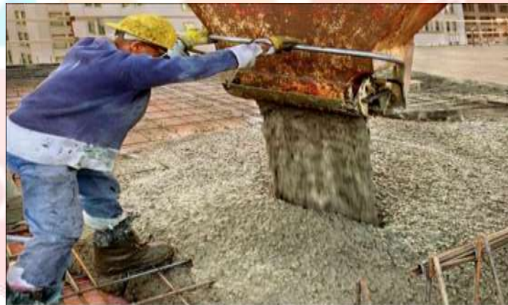
Fig.3 Casting of Precast Elements
