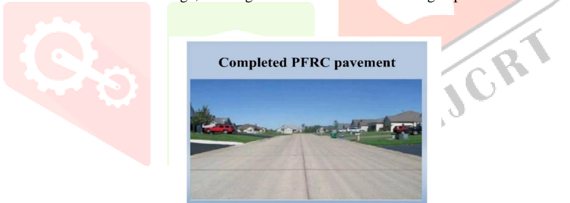
Fig no. 09 Completed PFRC pavement
