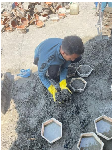
Fig 6: Pouring the mix in mould
