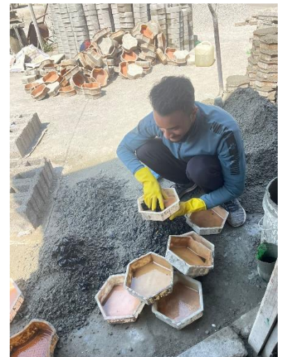
Fig 6: Oiling the paver block mould
