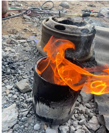
Fig 2: Heating Bitumen
