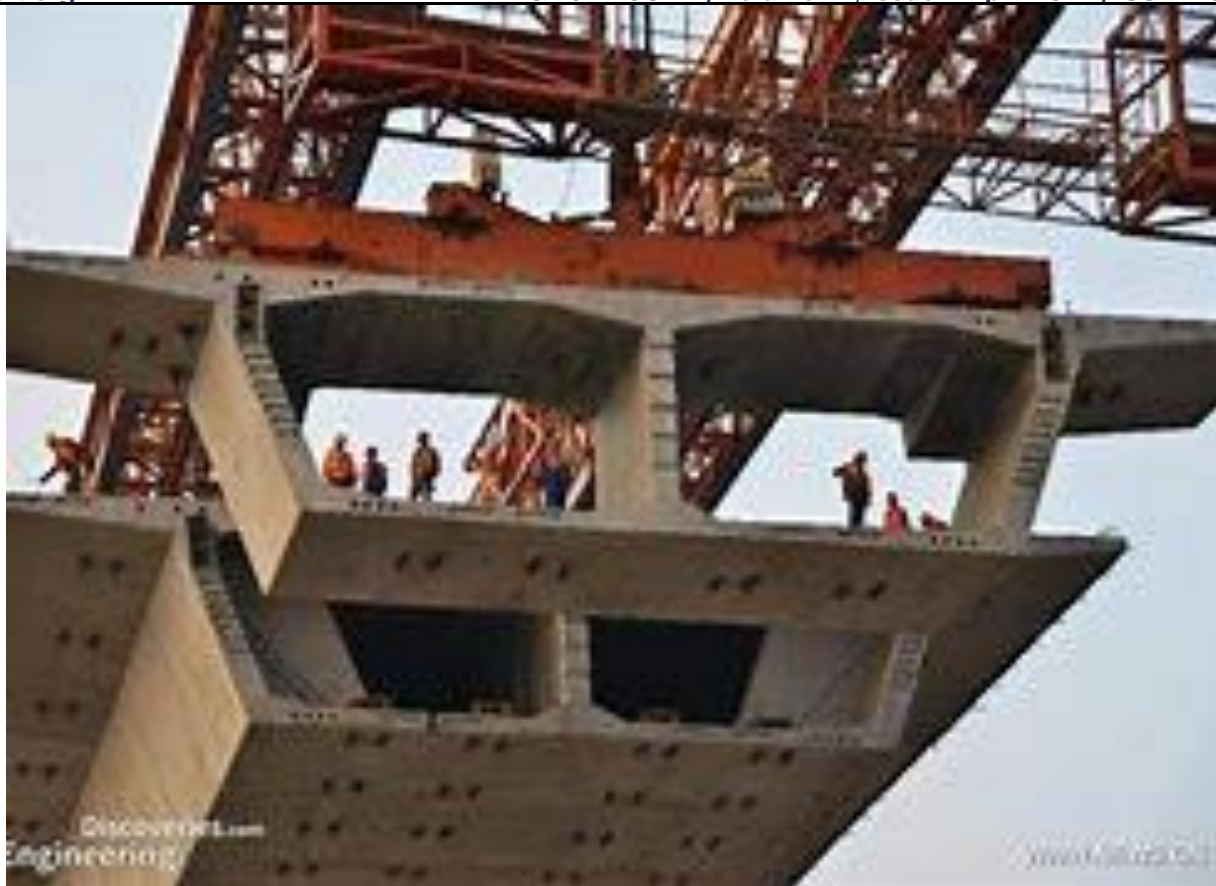
Fig 1.1 Typical Box Cell Section
