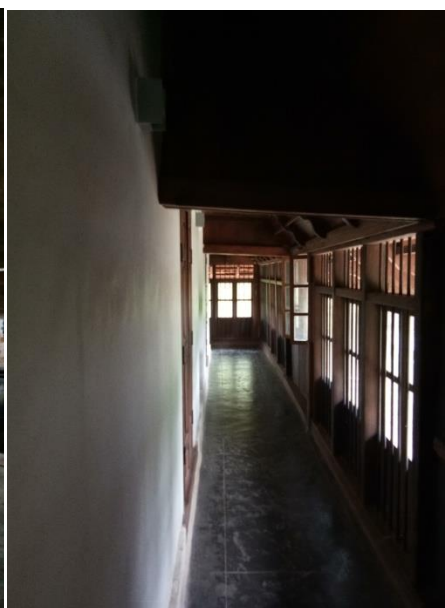
Figure: 15 – first floor corridor
