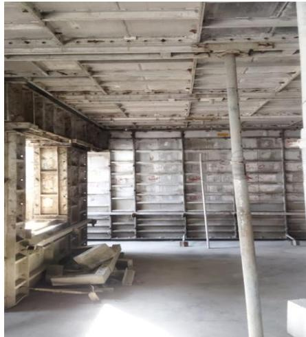
Fig No. 1 Aluminium Formwork
