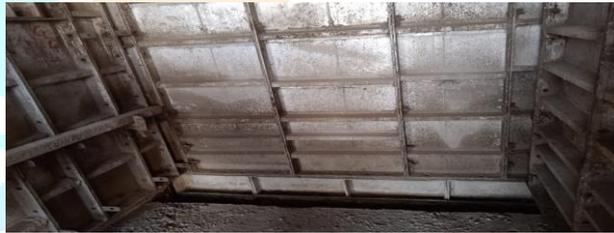
Fig No. 3 Aluform Fixing
