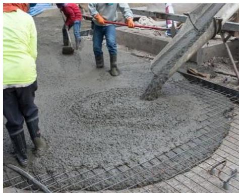
Fig No. 4 Concrete Pouring
