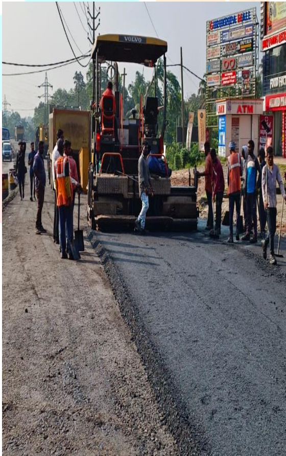
Fig.No. 14: DBM with 20% RAP laying at Site
