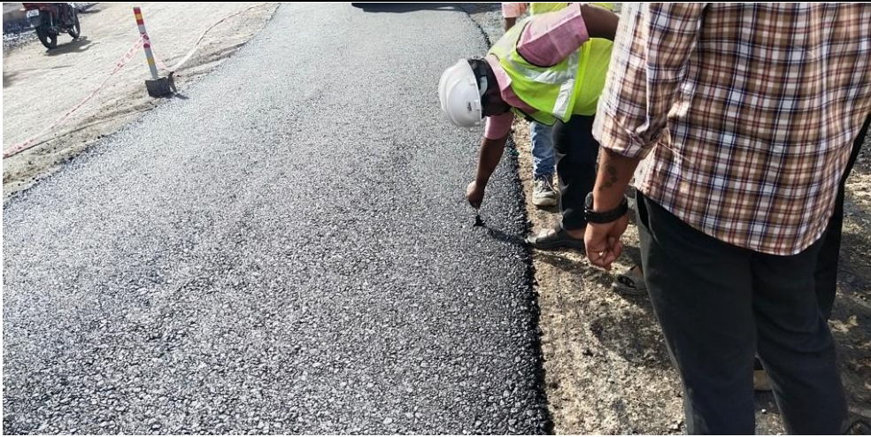
Fig.No.11: BC with 8% Plastic Fibre laying for 2.5 km stretch
