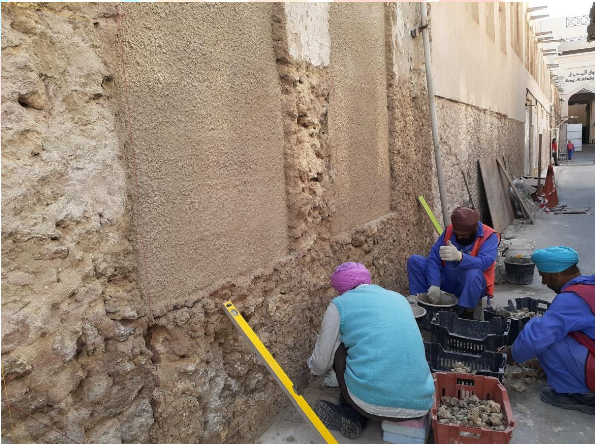
Fig.2. Removing of pre-existing plaster.
