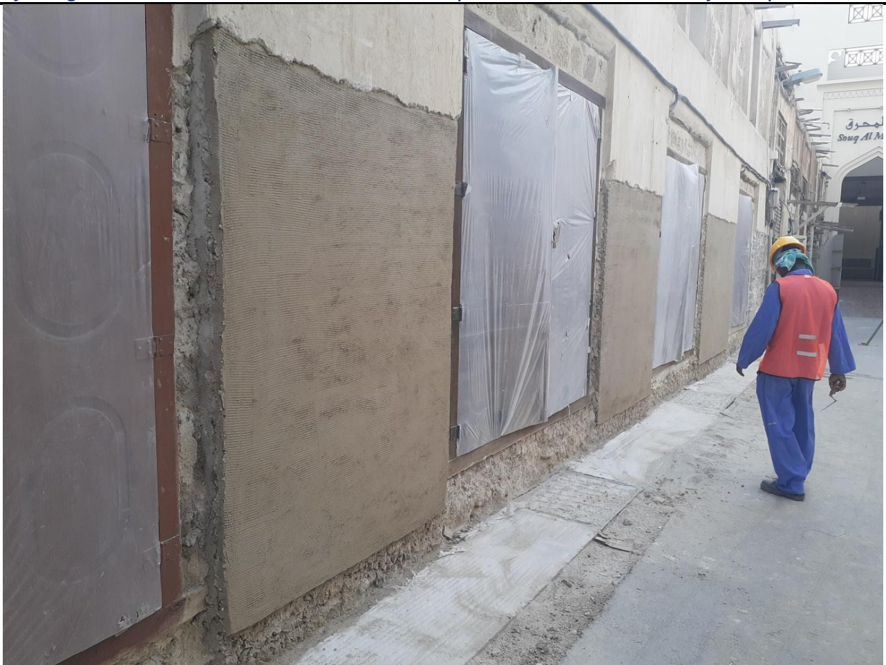
Fig.4. After the structural conservation of the walls.
