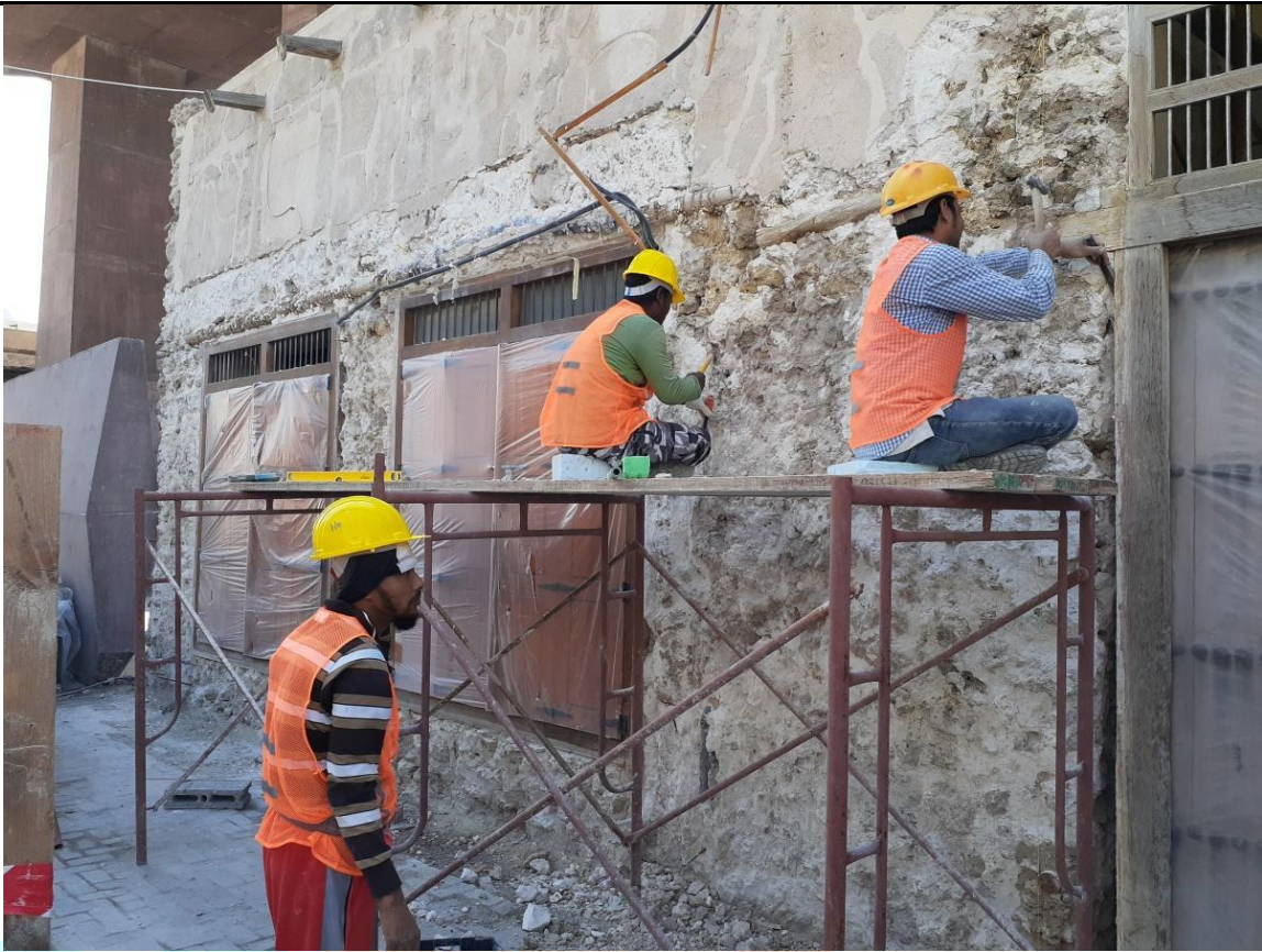
Fig.2. Removing of pre-existing plaster.
