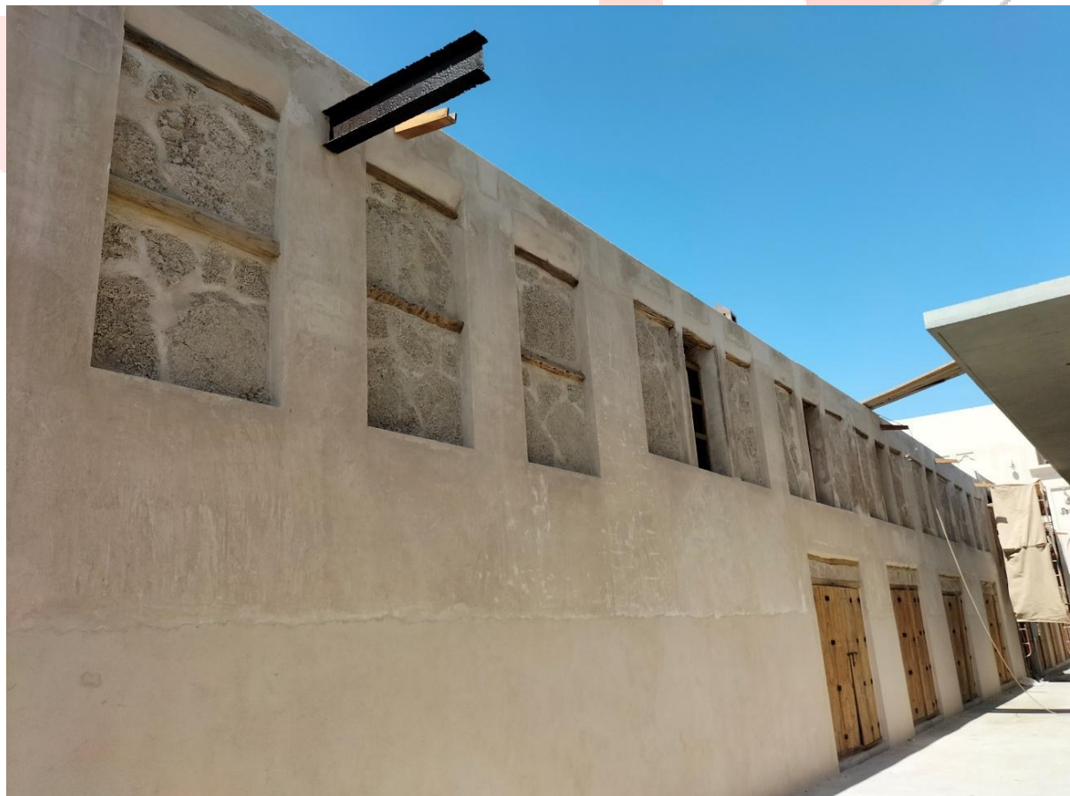
Fig.5. Final view of the structure after conservation.
