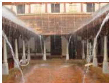
Figure 4: Courtyard View to Harvest Rainwater
