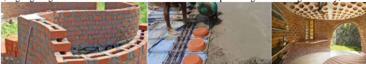
Figure 10: Construction Techniques Followed
