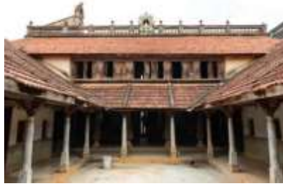
Figure 5: View from the Courtyard: Linking with Nature
