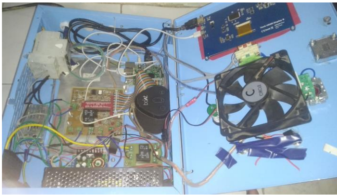
Fig. 21. Internal arrangement of Modules
