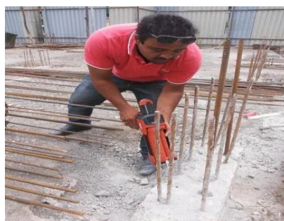
Fig2. Application of epoxy Rebar
