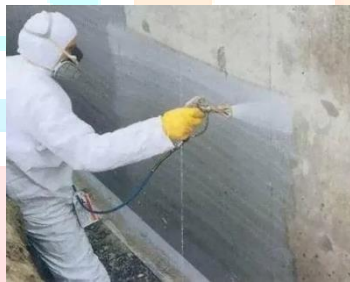
Fig3. Epoxy used in water tank wall
