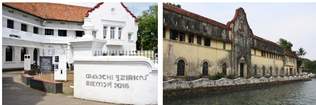
Figure 5(left): Entrance of Aspinwall House featuring the sloping roof with Mangalore tiles, deep eaves and semi-circular arches. Figure 6(right): The sea-facing facade of Aspinwall House. Source: (MASTERS, 2017)
