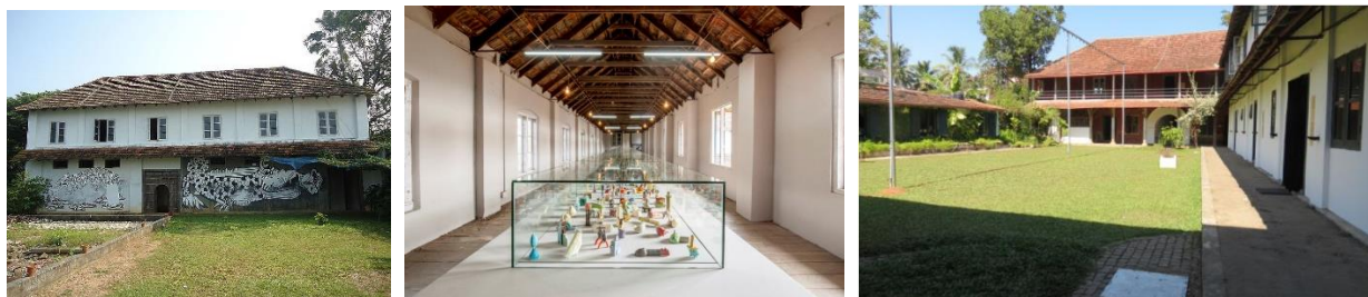
Figure 13(left): Exterior view of Pepper House Figure 14(middle): Interior view of Pepper House exhibiting the traditional wooden post beam structure Figure 15(right): Courtyard of Pepper house in nadumuttam style. Source: (Siji, n.d.)
