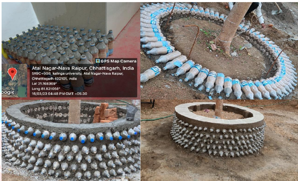
Figure No. 1: Bottle Brick Construction
