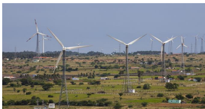
Fig3. Land and infrastructure [19]
