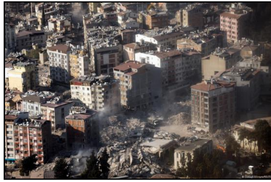
Figure 1: Damages of Structures due to Earthquake Occurred in Turkey
