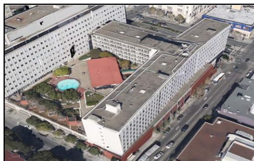
Figure 2: Re-entrant corner Building
