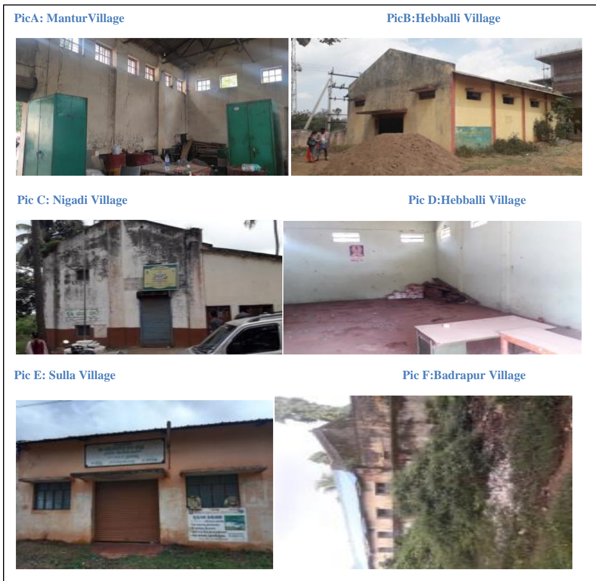
Picture 1: Status of Rural Godowns in Selected Villages of Dharwad District
