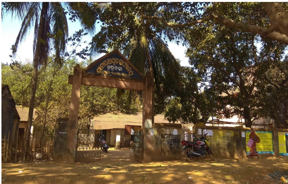
Figure 3.1: Gram Panchayat Office
