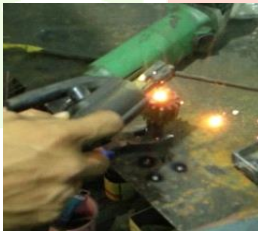
Fig: 14 joining of pipes Arc Welding
