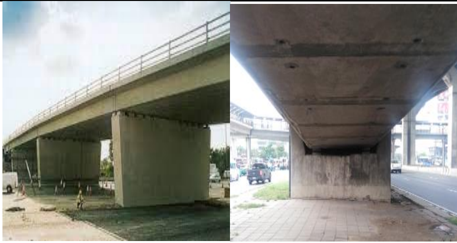
Figure 1:- Showing Slab bridges
