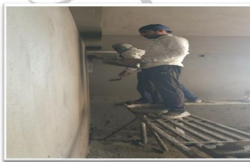
Fig. 8. Plaster Work
