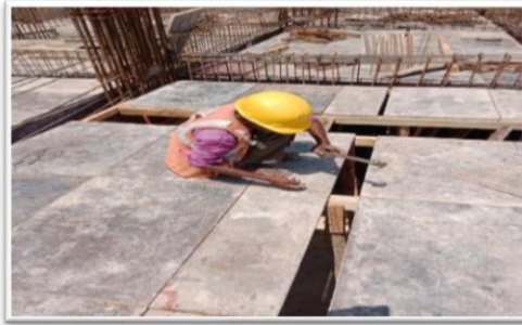
Fig. 4. Shuttering Work
