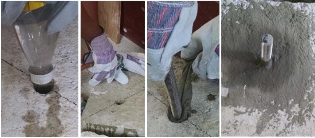
Figure Test Series 0c Installation Photos.
