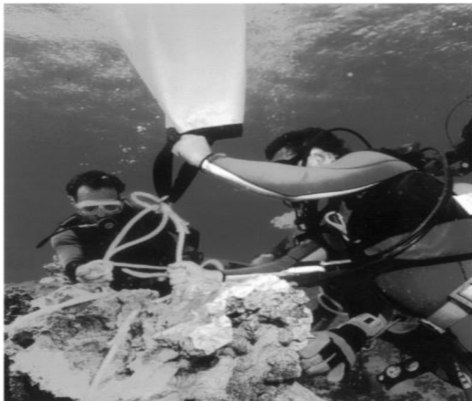
Fig-5 Lift bag, moving George Town, Grand Cayman large boulders, Maasdam restoration, Soto's Reef, , British West Indies. Photo credit: T. Fulton.
