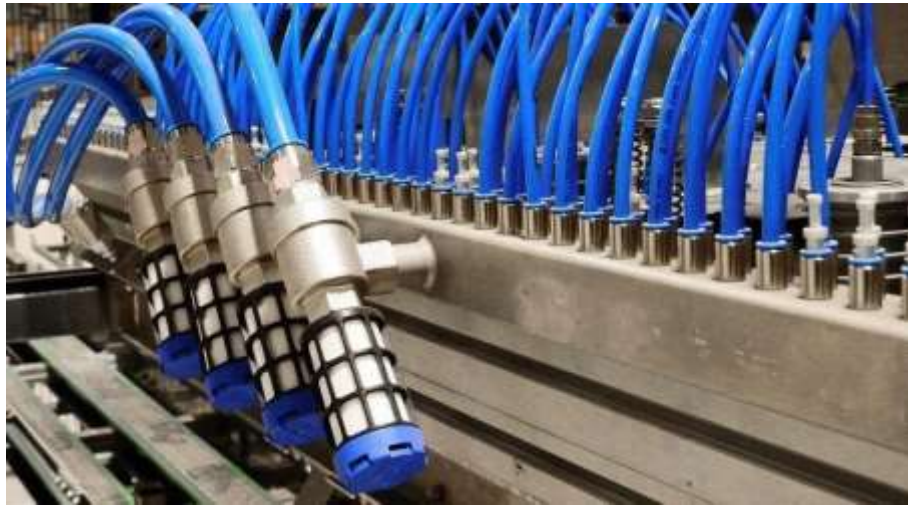
Fig (1.6.1) pneumatic hoses and tubing
