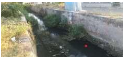
Open drainage channel
