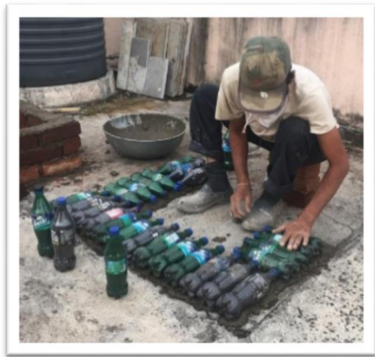
Figure 4: photograph of bottle brick masonry
