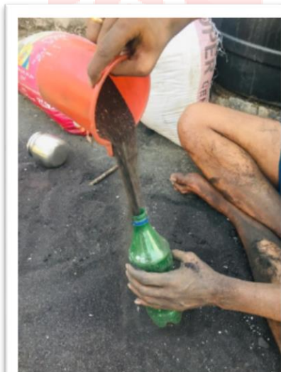
Figure 2: photograph of filling of waste foundry sand in PET bottle
