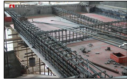
Fig1.9: beam-beam joints
