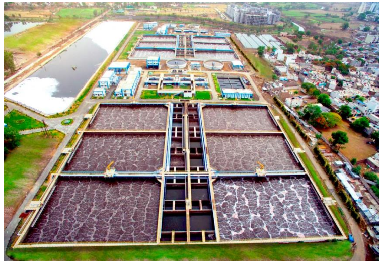
Figure 1: Photographic view of Sewage Treatment Plant, Kabitkhedi, Indore
