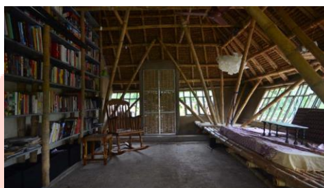
Figure 2.3 and Figure 2.4 First floor of the Baruipur House supported on bamboos (Source: downtoearth.org.in)
