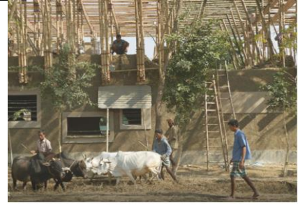
Figure 4.2 Upper floor walls are made up of bamboo and lower floor using Cob technique (Source: Arch Daily)
