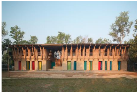
Figure 4.1 Handmade school in Bangladesh (Source: Arch Daily)
