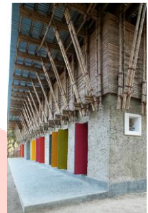
Figure 4.6 Bamboo frame structure (Source: Arch Daily)
