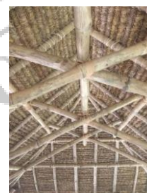
Figure 3.3 Balinese- style thatch roof (Source: downtoearth.org.in)
