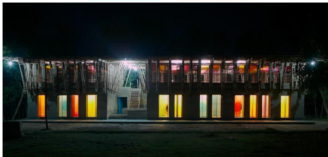
Figure 4.5 School at night with contrast ceiling color with help of saris (Source: Arch Daily)
