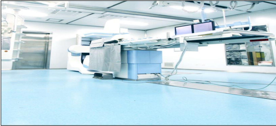
Figure.7 Polyurethane concrete flooring
