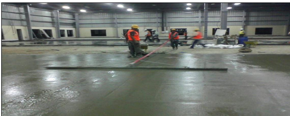
Fig. 3 Laying process of FRC flooring
