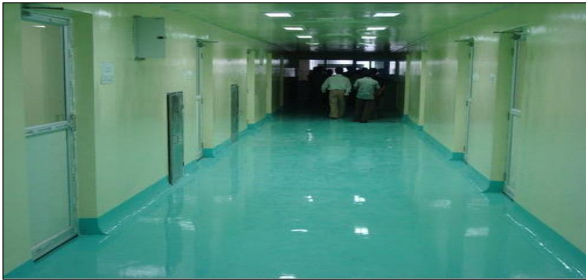
Figure 8 Epoxy flooring
